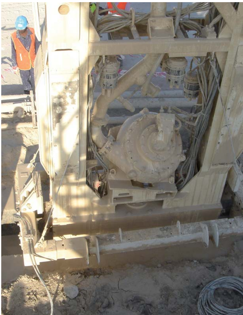
a) SOILMEC 'Tiger' series hydromill (hose drum design)
